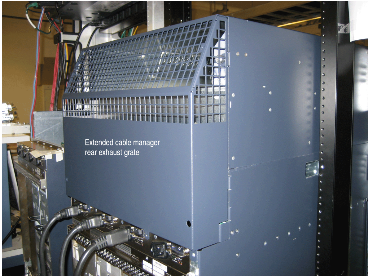
Figure 102: Installing the New Rear Air Exhaust Grate
