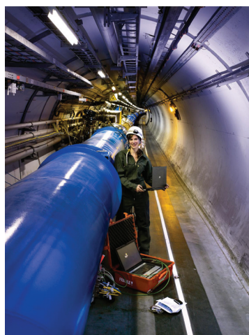
Engineers check the electronics of the cryogenic instrumentation under a dipole magnet. ©CERN.
