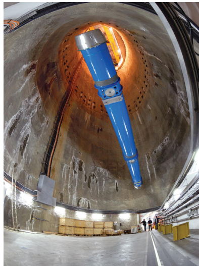
The last of 1,746 superconducting magnets is lowered into the LHC tunnel via a specially constructed pit. This 15-m long dipole magnet is one of 1,232 dipoles positioned around the 27-km circumference of the collider. Dipole magnets produce a magnetic field that bends the particle beams around the circular accelerator. ©CERN.
