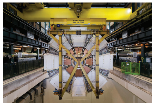
Engineers lower the second small wheel down the 100 m shaft into the ATLAS cavern at the Large Hadron Collider (LHC) at CERN in Switzerland. ©CERN.
